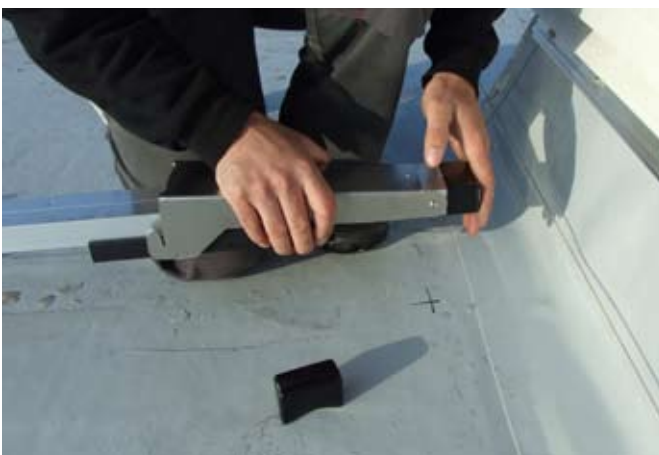
Place end caps on rail ends
