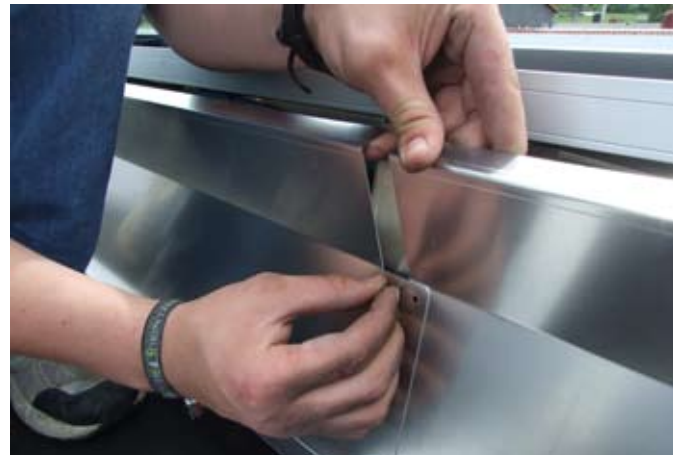
Place screw in the slot
