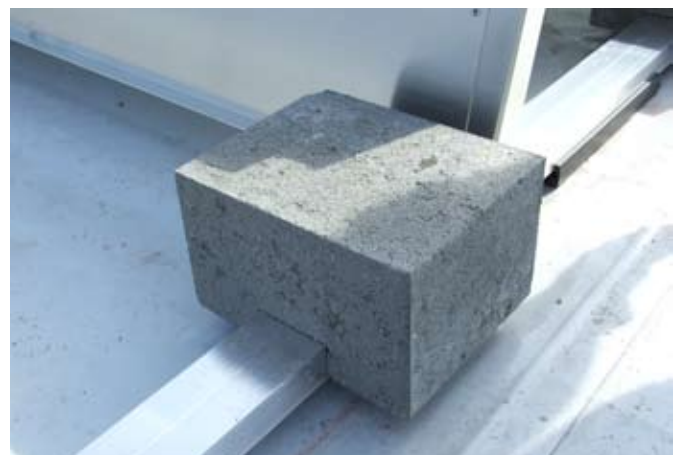
Place ballast according to plan
