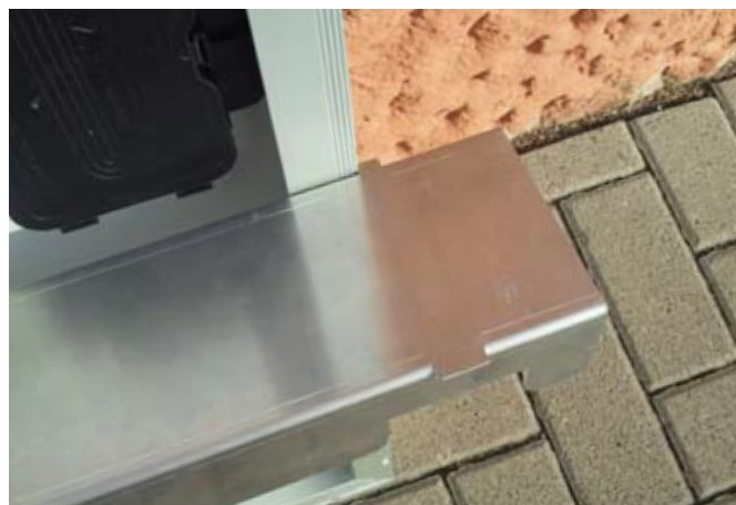
For justification press small catches to both module frames.
