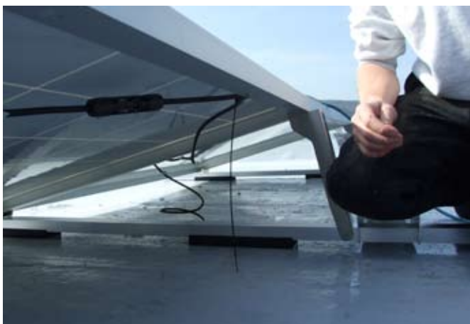
Carefully tighten cable tie
