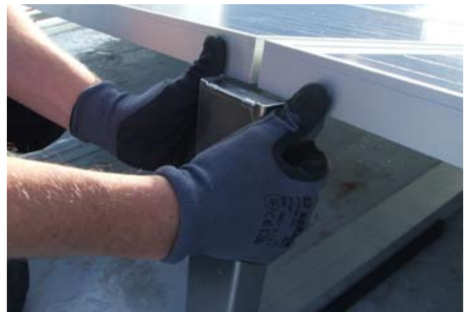
Lift next rear bracket into position
