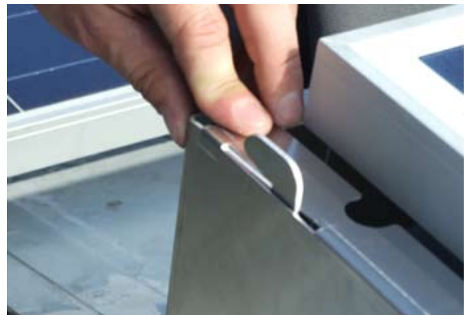
Hook groove into rear bracket
