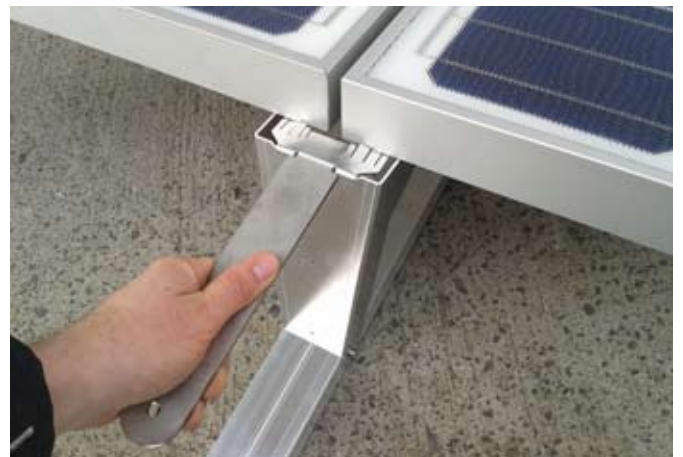
Bend up securement tabs slightly
