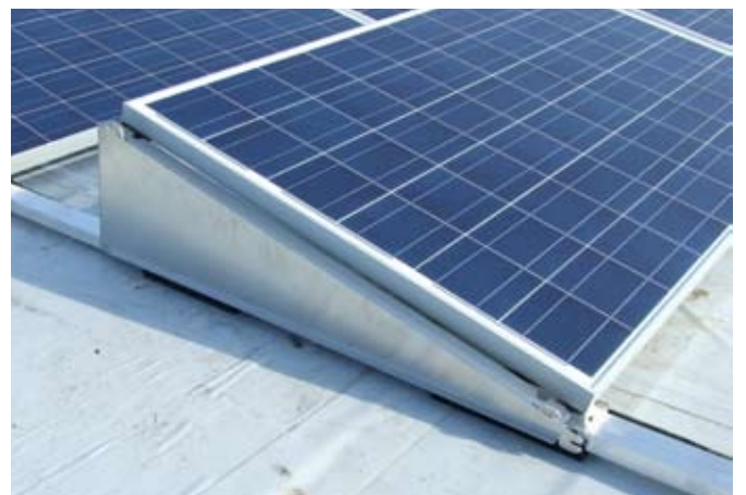
Side sheet installed
