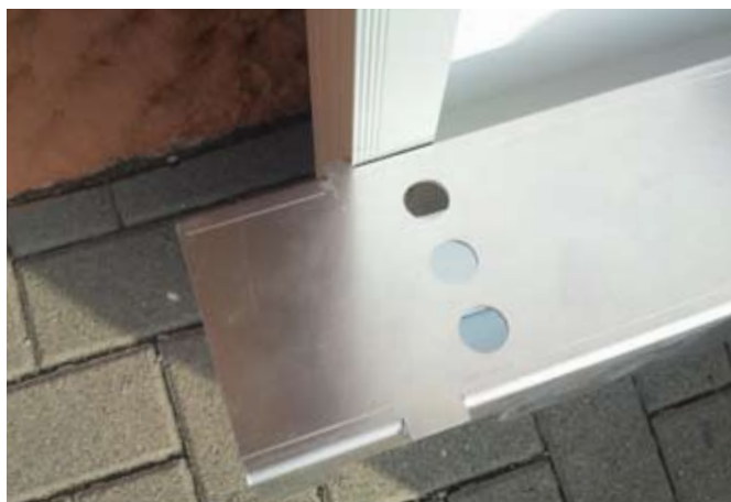
For justification press small catches to both module frames.
