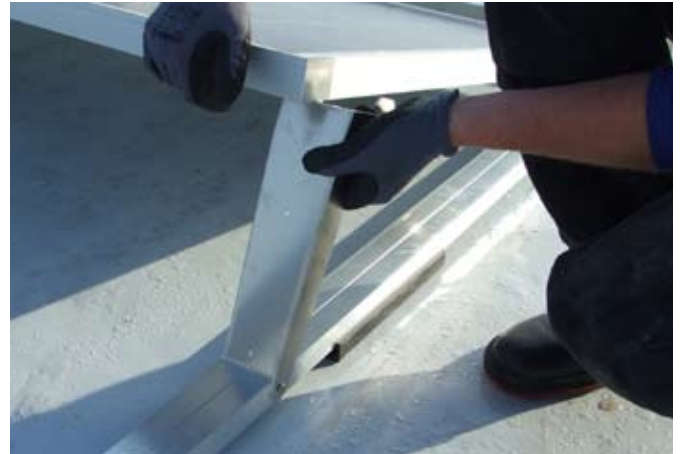
Lift rear bracket into position
