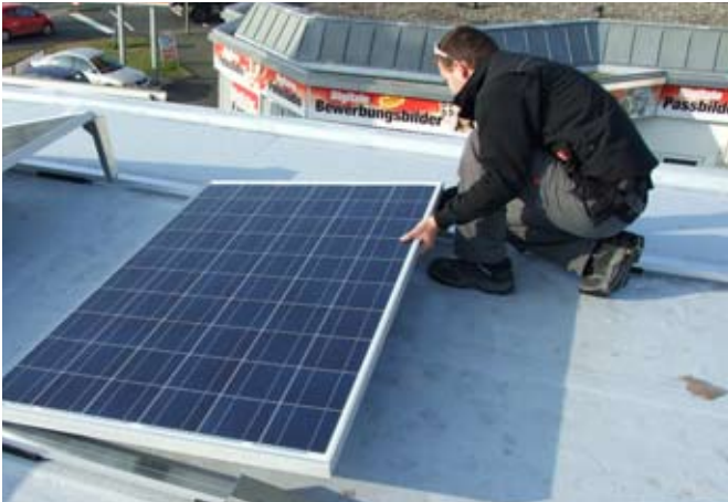
Lift module to target inclination
