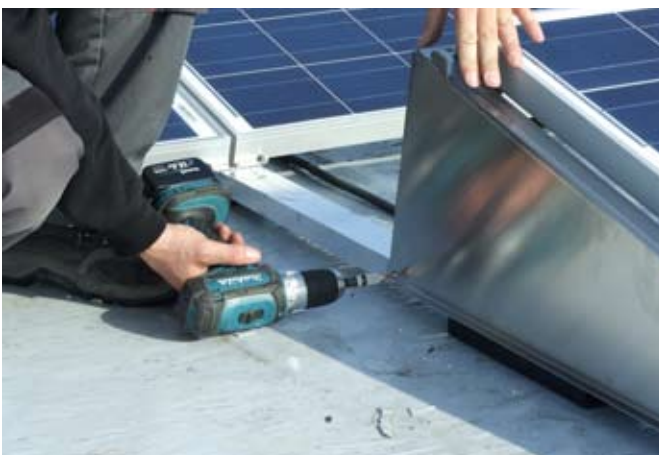
Secure with screw - end bracket
