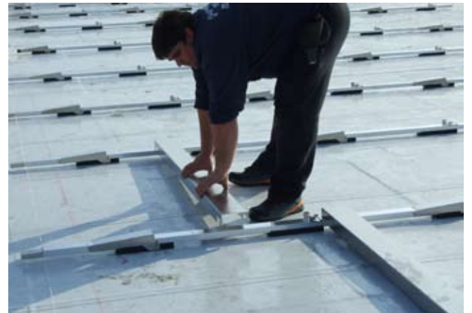
Align rails to string line
