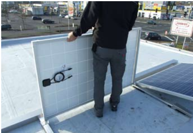
Place module upright on the rails
