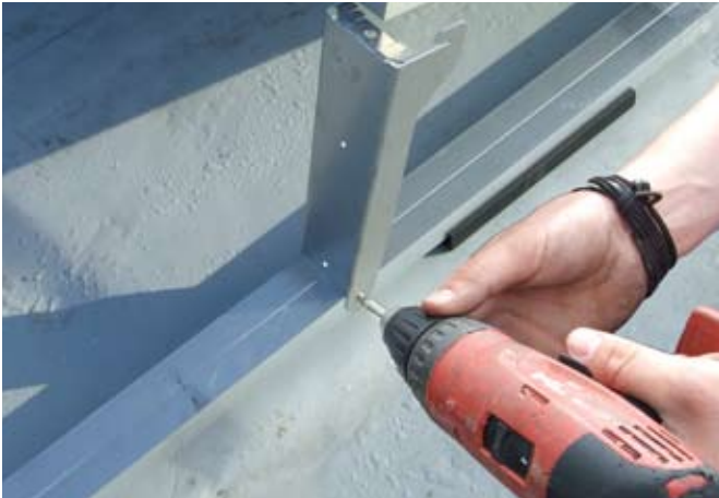
Loosen screw at end bracket
