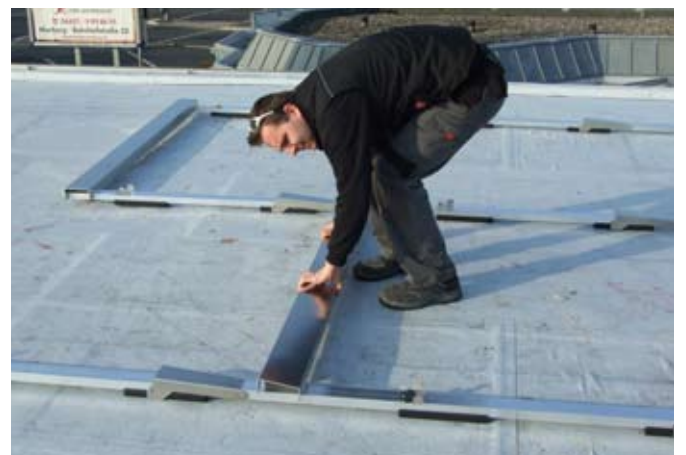
Fixed width set up with layout bar in the south behind rear bracket
