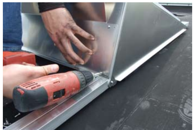
Finally screw sheets at the bottom
