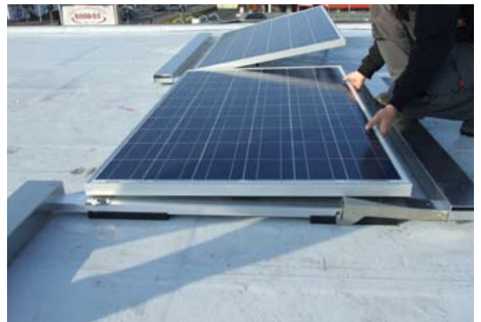
Apply pressure on layout bar (knee)
