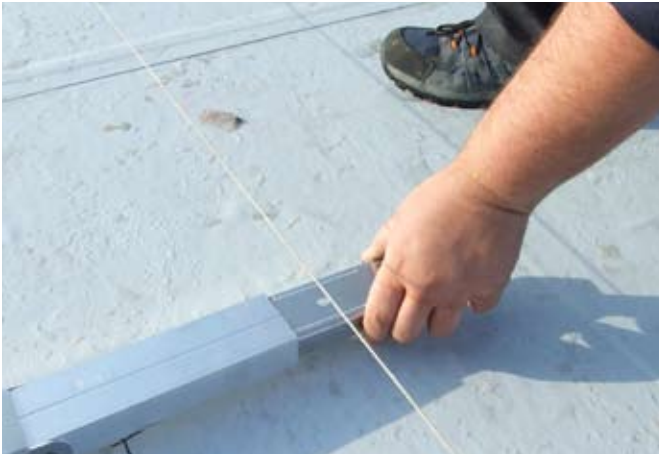
Insert rail connectors
