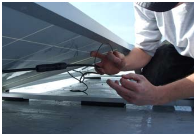
Insert cable tie into frame hole
