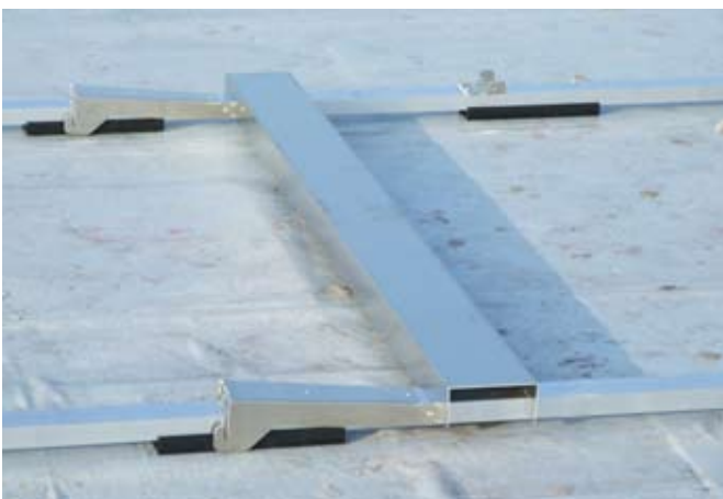
Fixed width set up with layout bar in the south behind rear bracket
