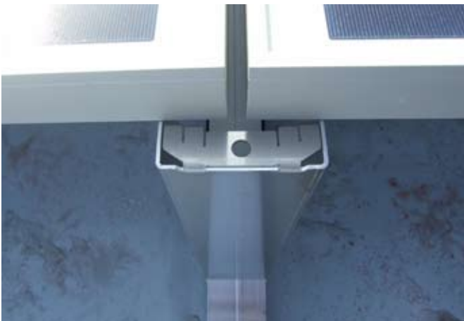
Check bracket layout and align
