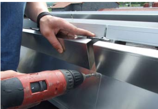
Secure sheets into rear bracket
